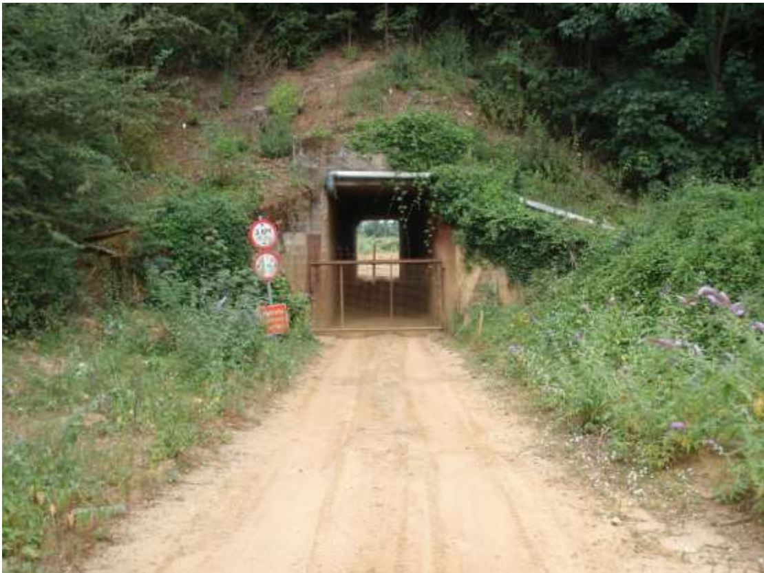
Plate 21. Tunnel located on PDA
