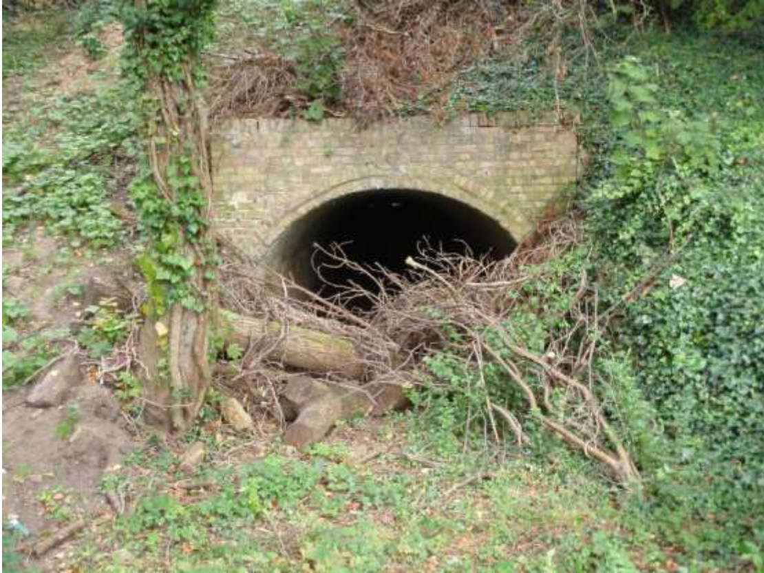
Plate 20. Tunnel located on PDA
