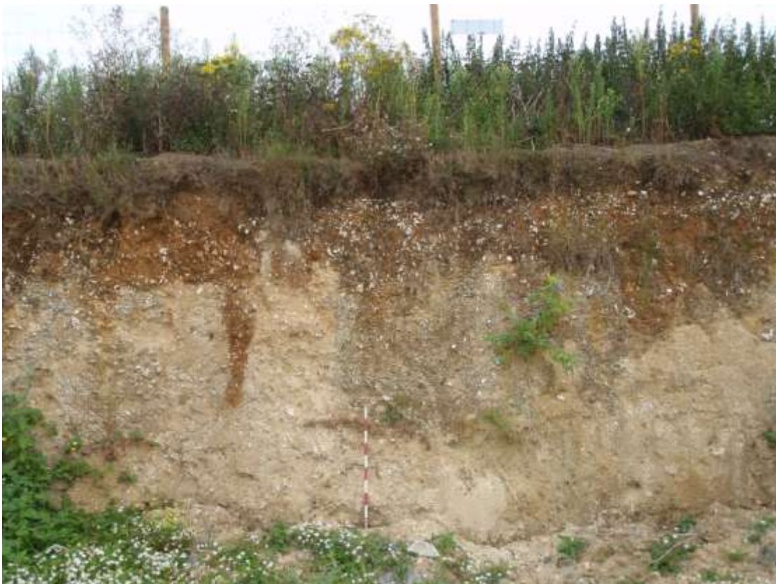
Plate 19. Typical quarry face section on north side
